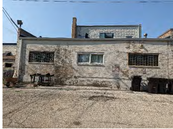
Photo 2: Lintels at rear elevation
