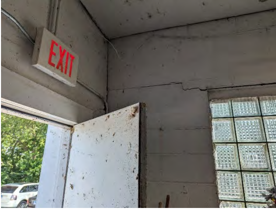
Photo 5: Interior view of NW corner
