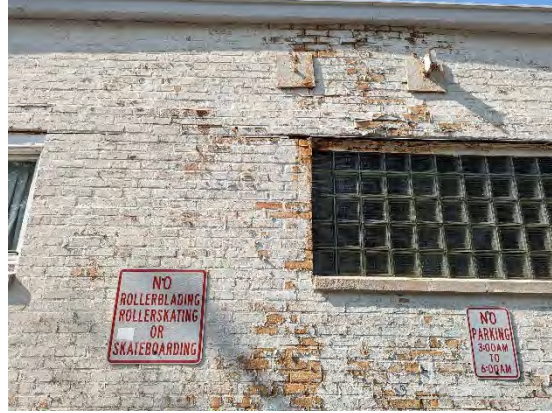
Photo 10: Steel plates at rear wall
