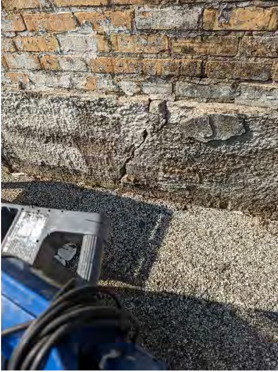
Photo 9: Foundation cracking
