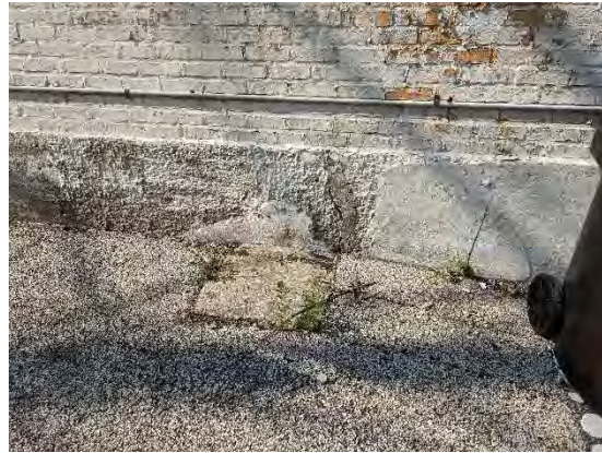
Photo 4: Foundation cracking
