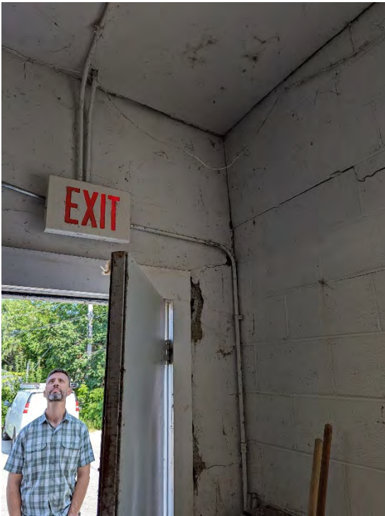
Photo 7: Interior view of NW corner
